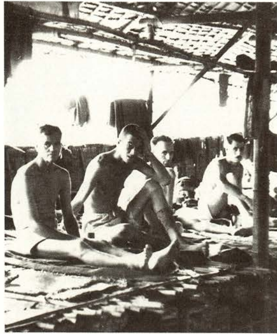
Australian prisoners of war used in the building of the Burma–Thailand Railway. Thousands of Australians endured the horrors of Japanese imprisonment but they had a better survival rate than other Allied prisoners. This photograph of the interior of a typical 100-metre atap-roofed hut illustrates the cramped sleeping space for each man – usually not more than 76 centimetres.
